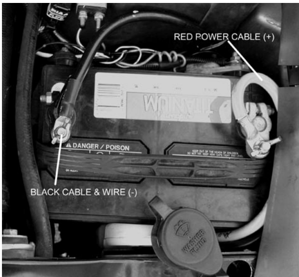
2-14: Complete Wiring to Battery
